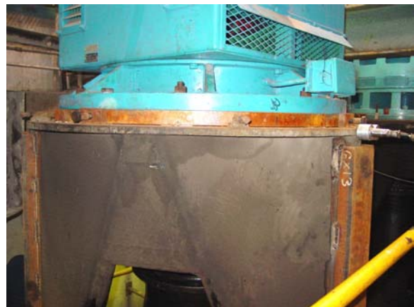
Figure 5B • installed stiffeners
